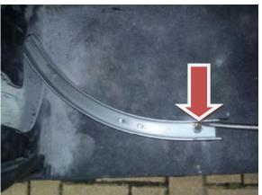
Place the curved piece of track onto the template you marked on the floor of the step well earlier, making sure it is firmly against the front of the stairwell. Using a self drilling screw fix the track to the floor at the rear most point first, taking great care to be as accurate to your template as you can. You will need to place the screw as far to the inside of the track as you
